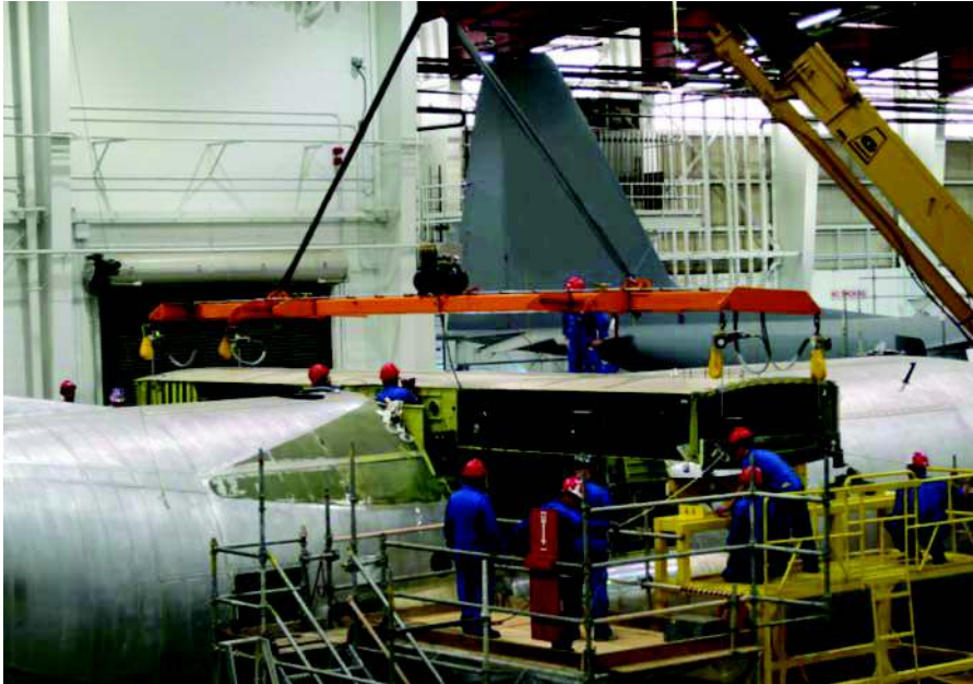
Figure A-3 Positioning a C-130 Centre Wing
